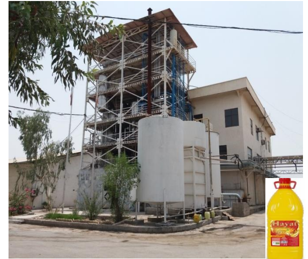
Hayat Hormozgan co. Industrial park of Bandar Abbas
